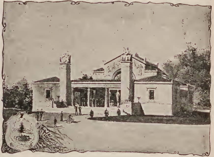
VERMONT STATE BUILDING.
